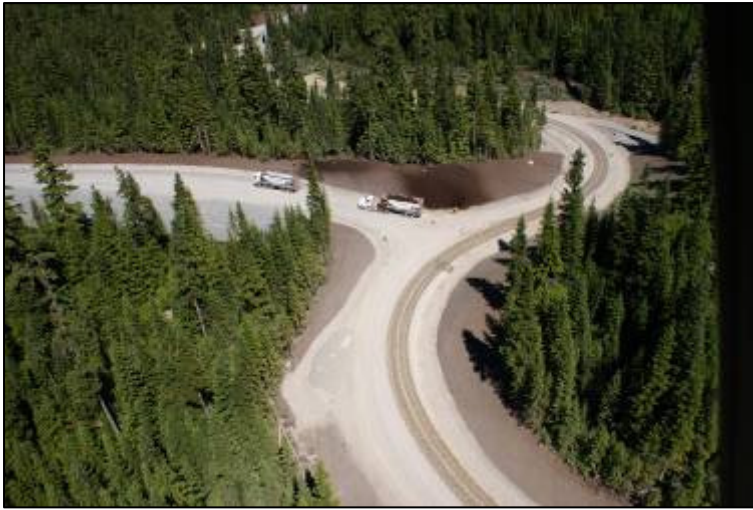
Pneumatic installation and Terraseeding™ of compost blankets for erosion control on soil slopes throughout venue
