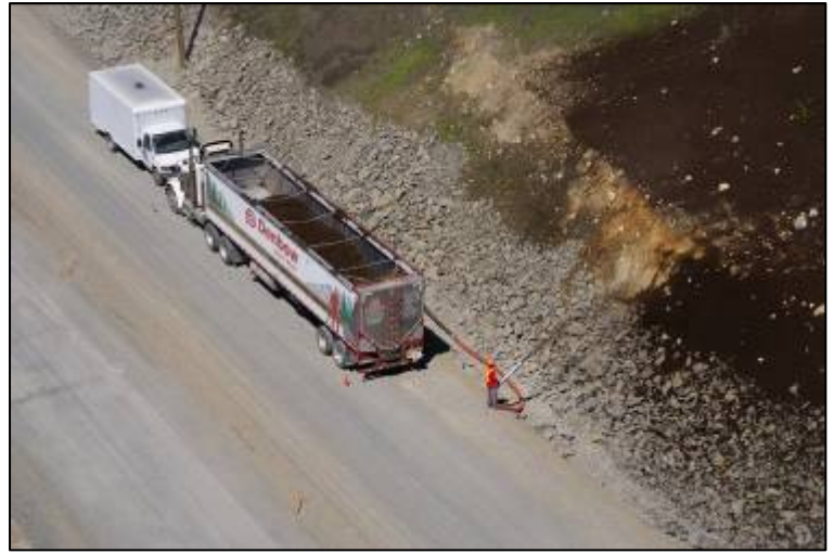
Pneumatic installation and Terraseeding™ of compost blankets for erosion control on soil slopes throughout venue
