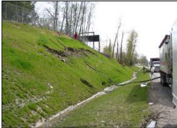
Problem: Slope had been hydroseeded and failed multiple times.
