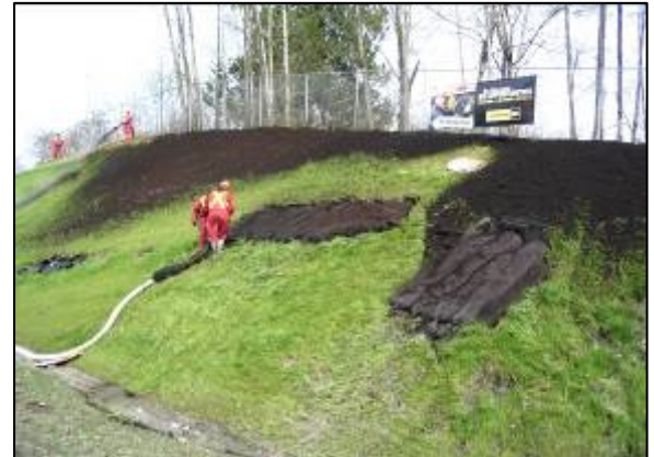
Denbow's solution: Apply FilterSoxx™ to fill holes in slope and EcoBlanket® for revegetation
