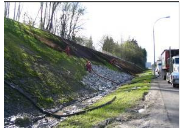
Denbow's solution: Apply FilterSoxx™ to fill holes in slope and EcoBlanket® for revegetation
