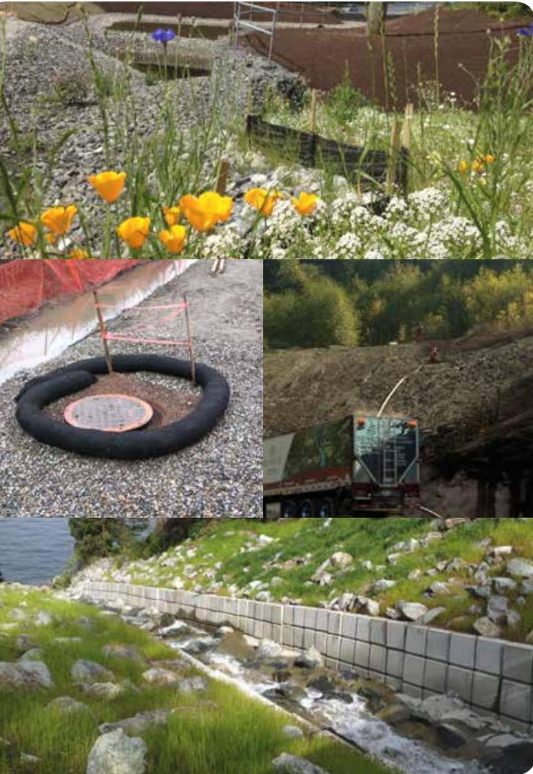
Compost filter socks provide a three dimensional filter that retains sediment and other pollutants (e.g., suspended solids, nutrients, and motor oil) while allowing the cleaned water to flow through.
