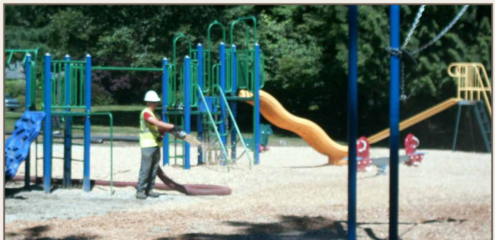
PlayChip installation with blower truck
