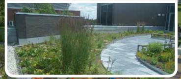
Green roofs retain rainwater, and act as natural filters for any of the water that happens to run off the building.
