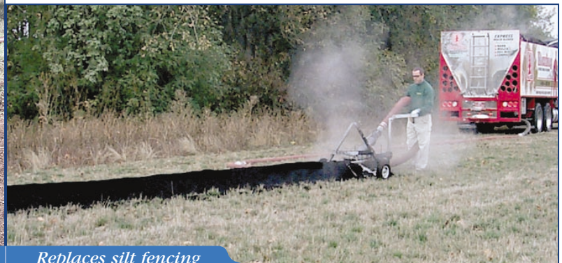
Replaces silt fencing
