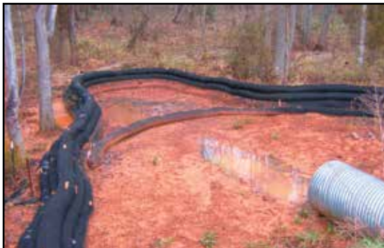
Use at Basin Outfall.
