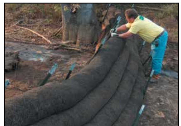
Stacking Method for Sediment Traps.
