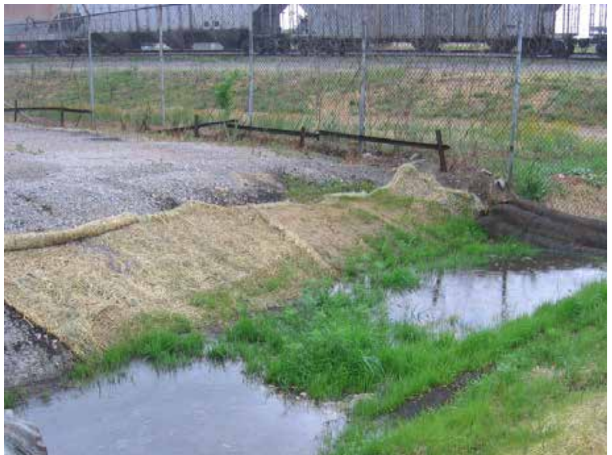
Figure 2. Filtrex ® Filtration system was installed April 20th, 2007, to evaluate their performance on chemical oxygen demand (COD), total suspended solids (TSS), and oil and grease in the storm water effluent from CWS Outfall #2.
