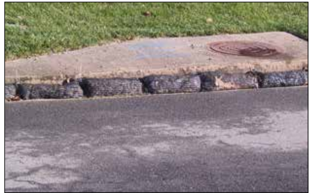
Typical rock bag installation for inlet protection
