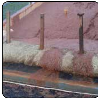
Fig. 6: 20" Straw Wattle (70% Removal Efficiency)
