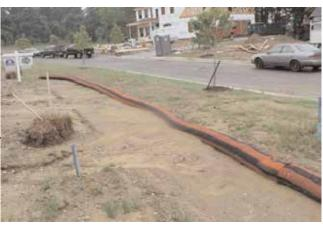
Filtrexx Soxx<sup>™</sup> (SiltSoxx<sup>™</sup>, InletSoxx<sup>™</sup>, DitchChexx<sup>™</sup>) are three
